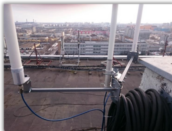
FIG. 5B EXAMPLE OF CORRECT ANTENNA MOUNTING
