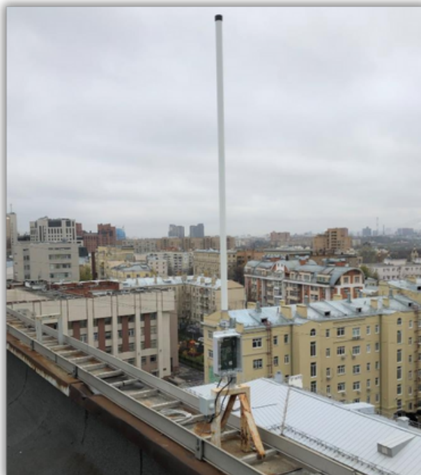
FIG. 5A EXAMPLE OF CORRECT ANTENNA MOUNTING
